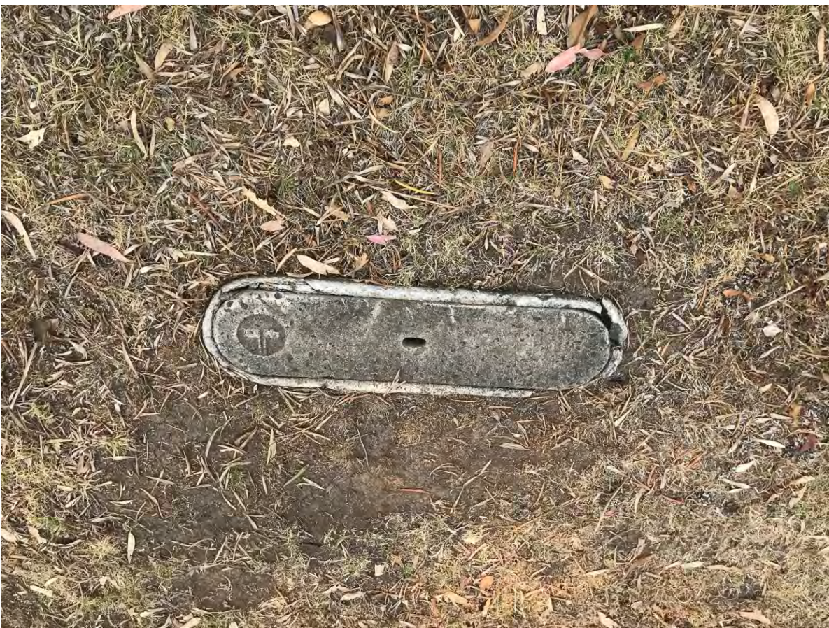
Photograph 18: a Telstra telecommunications pit potentially containing asbestos cement observed within public space within the alignment
