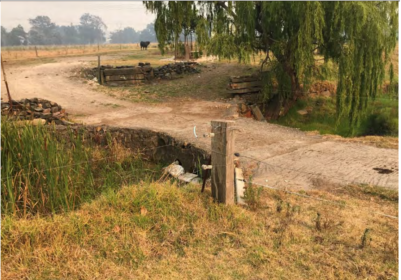
Photograph 11: a creek crossing over Hazleton Creek observed within Lot 1 in DP559819, constructed of rock, concrete with several concrete culverts observed
