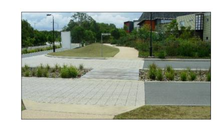
**21.** Avoid displaying shareway information and other bicycle advisory signs on poles as these are susceptible to vandalism and will leave pedestriar signage should be displayed via path templates of on path constrictors. Signage should be provided i relation to access onto the off road SUP network, to signify to entering users it is a shared facility. Signage should be provided on the SUP network at reasonable intervals to signify to users it is a shared use facility.
