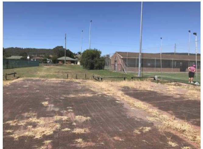
4. Kimbeth Crescent Car Park – Concrete paver parking in poor condition
